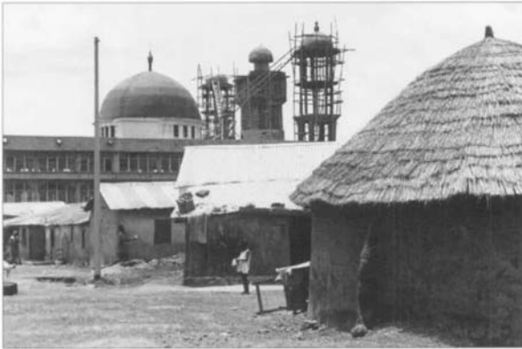
△ The mud-built men's rooms of a traditional compound contrast with the new central mosque being constructed in Tamale.
