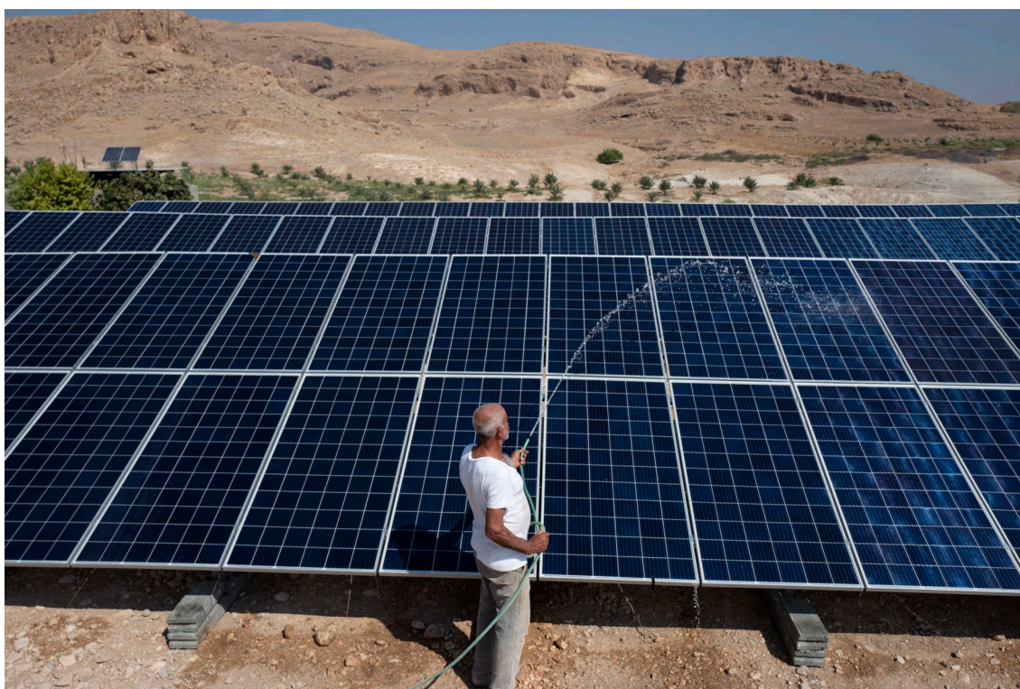
Ahmad is a date farmer in the Jordan Valley of the Occupied Palestinian Territory. He manages a date plantation and takes care of a new solar water system installed by Oxfam and partner Economic and Social Development Centre (ESDC). The farm has no access to mainland electricity so previously they were using high-cost diesel to power their irrigation pump. Now, the farmers have access to water at all times, their crops are healthier, and they are spending less money on fuel and more on their business and families. © Kieran Doherty/Oxfam
