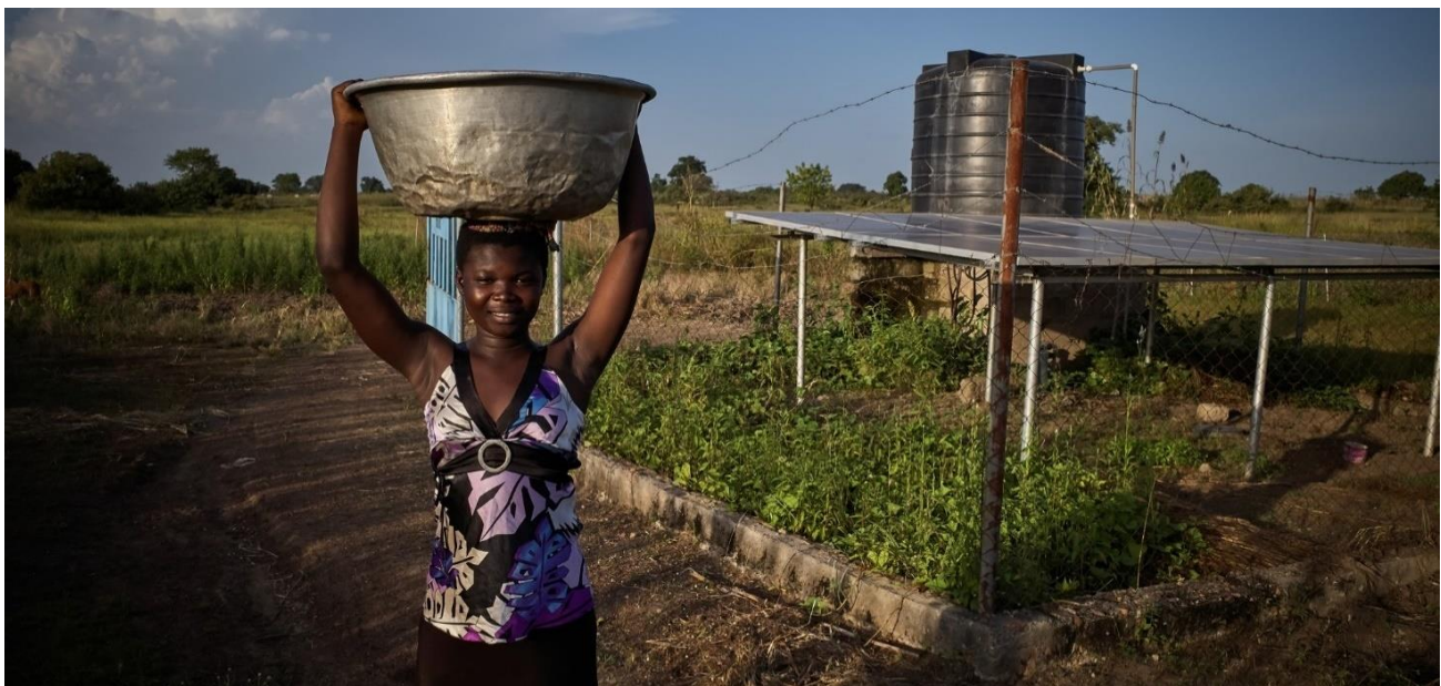
Photo: Collecting water from a solar powered water pump in the Garu District of Ghana.
