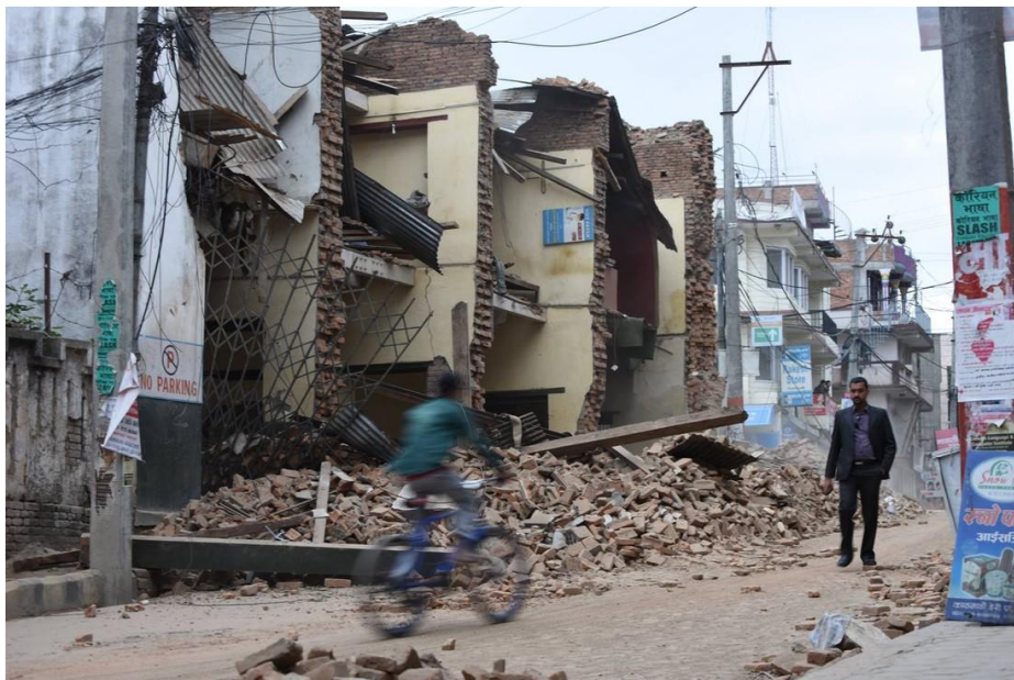
Homes were destroyed across Kathmandu. Photo: Shristi Rajbhandari
