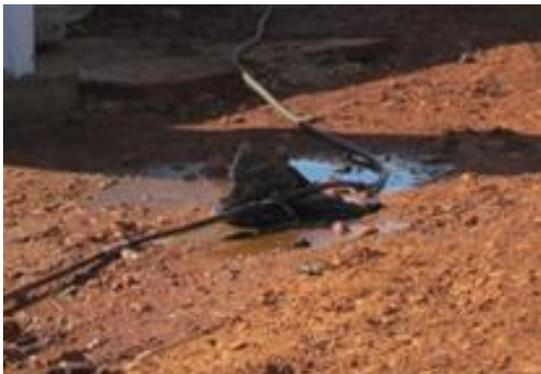
Another example of sanitary risk from local solution is provided by the mini distribution systems that residents create within the ITS, using plastic pipes laid on the ground. There is a risk of contamination as the pipes are not under constant pressure, they are likely to be punctured and they are often lying in contaminated stagnant water. See Figure 7 for an example.
