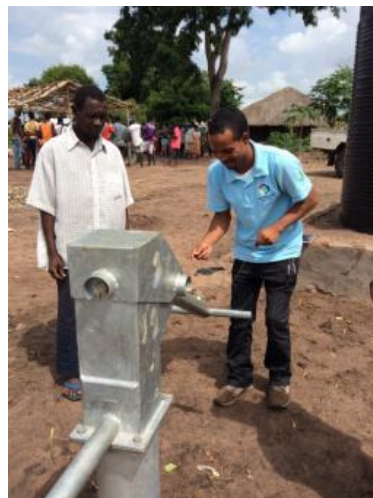
2. Carlos (Cecohas) on the right, maintaining a water fountain.
