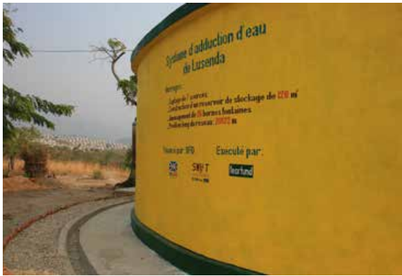
The gravity-fed water system at Lusenda
