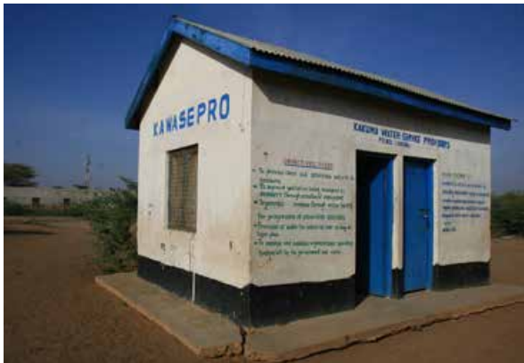
One of the water kiosks in Kabokorit
