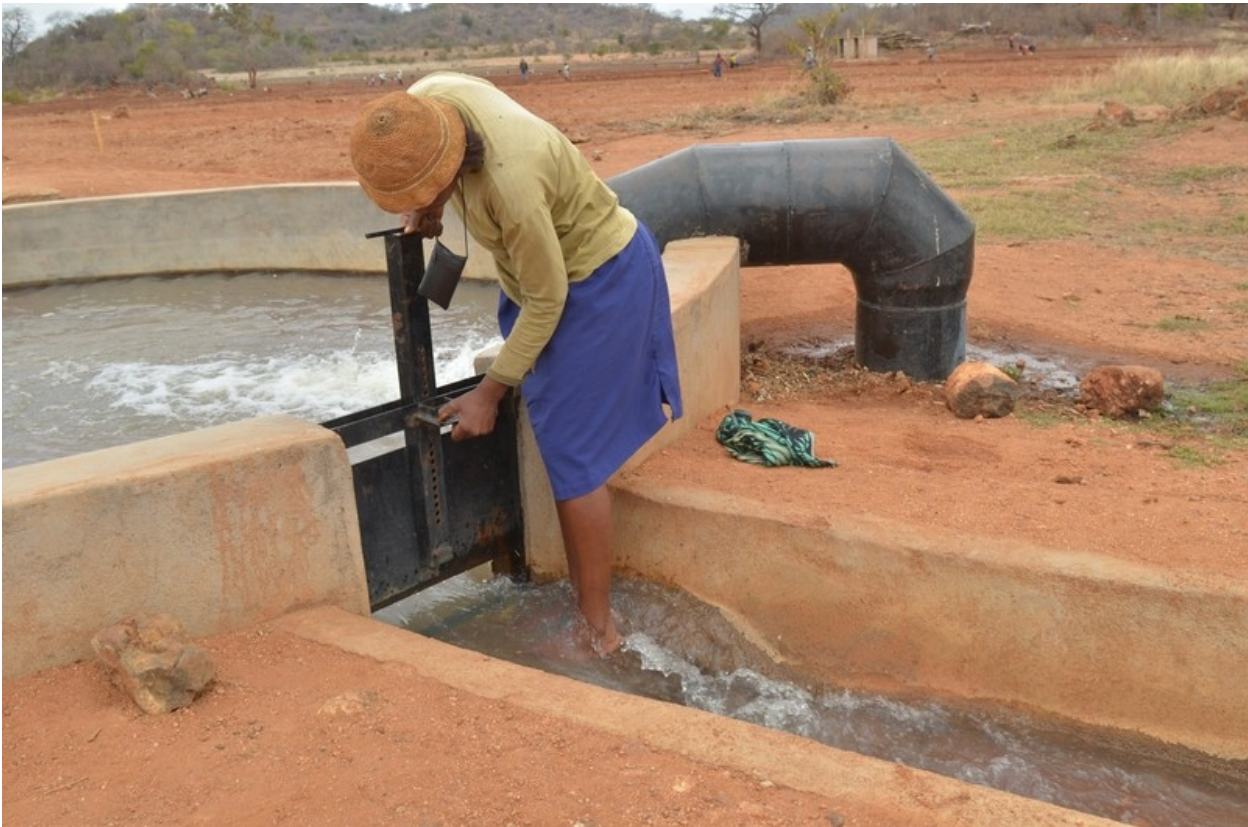
Ipaishe Masvingise opens and shuts sluice gates to direct water along the right channels to plot 64 where her first ever crop of wheat nears harvest. Ruti Irrigation Project, Gutu District, Zimbabwe, September 2011. Photo: Oxfam / Annie Bungereth.
