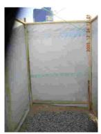
Washing slab for menstrual cloths inside a screened block and washing lines for drying the cloths.
