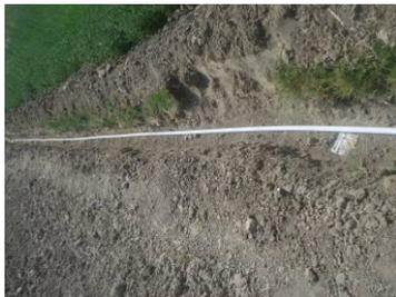
trench is dug from well pipe to pump head where the extension pipelines are laid & buried with soil. Un-skilled labour can be used to perform this work with close supervision and monitoring of a technically skilled person.
