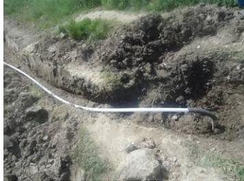
valve and the other end is connected to the bottom of the hand pump. Normally 1.25 inch dia pvc coil pipes are used as extension pipeline. A 12 inch wide and 12-24 inch deep (depend on the local situation)
