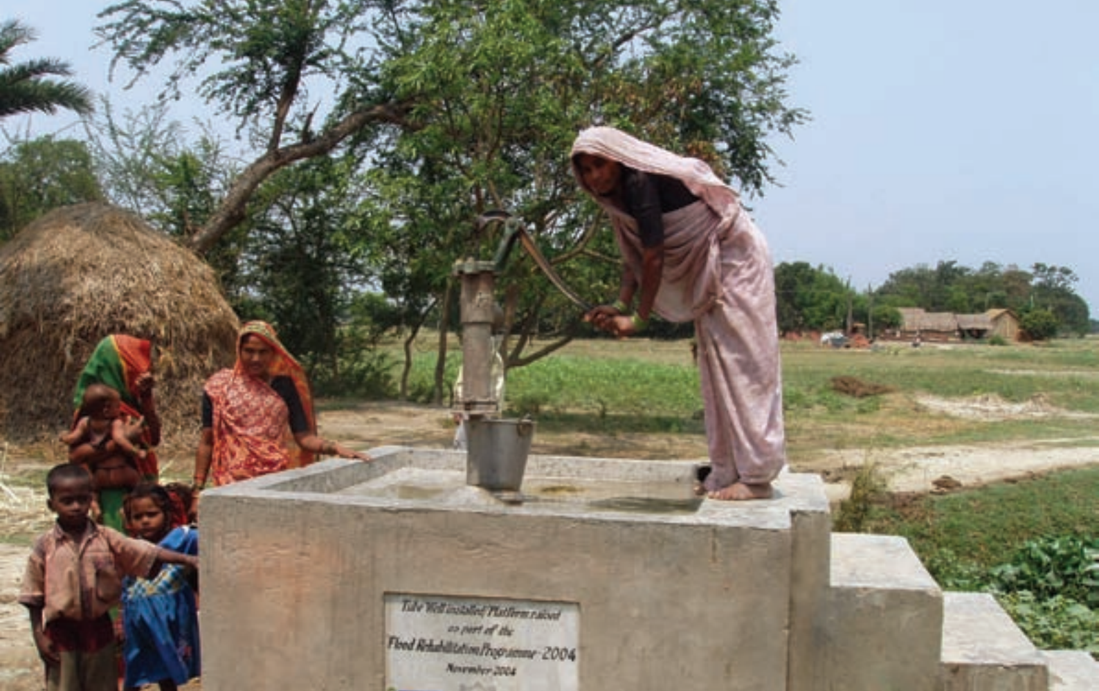
A woman demonstrates a raised tube well in the village of Harhi, India, installed as part of a flood rehabilitation programme. Photo: Gail Williams/Oxfam, 2005.
