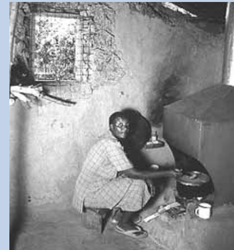
Reducing indoor smoke with a combination of an improved stove, smoke hood and eaves space in West Kenya (photo: Nigel Bruce/ITDG).
