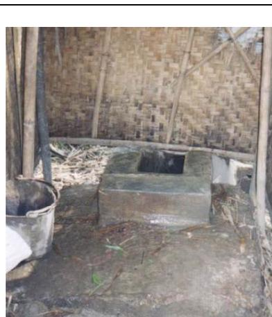
**Two vertical bamboo poles can be used for stability when squatting and for assistance when moving from standing to squatting position**
