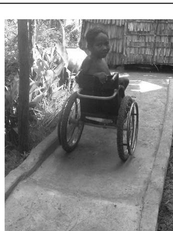
This concrete ramp provides a smooth access way for this child to the toilet. A kerb edge ensures the wheels of the wheelchair do not fall off the edge. (Jones & Reed, 2005)
