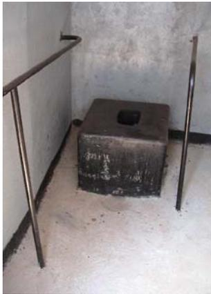
**Simple painted metal handrails fixed into the concrete floor and walls. GI / GS pipes and fittings or rolled hollow sections could be used**
