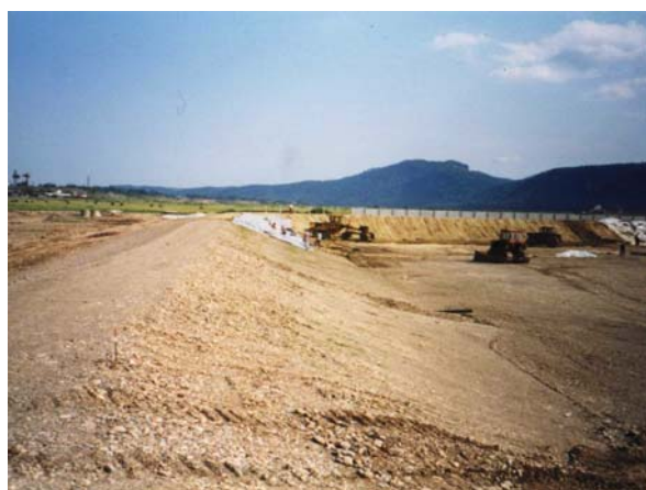
Figure: EU funded Engineered Landfill, Romania
