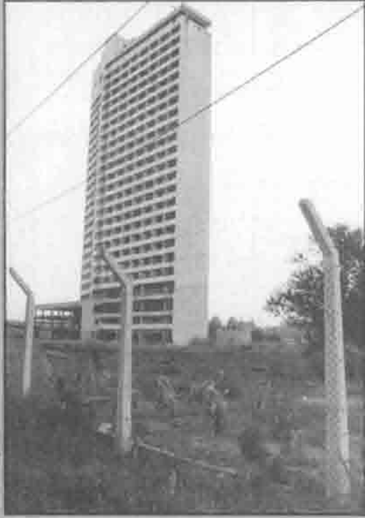
In 1975 the Portuguese poured concrete down the lift shafts and stole the plans of the partially completed Four Seasons Hotel on the Costa do Sol in Maputo. Today it remains a concrete shell.
