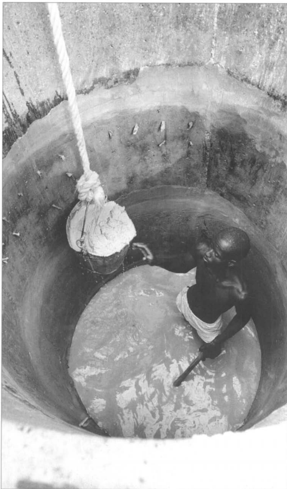
left An Oxfam-funded well under construction near Timbuktu
