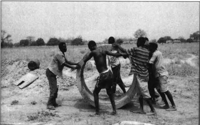
Kubore, Ghana. The regular inspection and checking of work are important.
