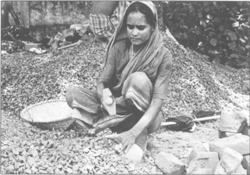
Working on the Road Maintenance Programme.
