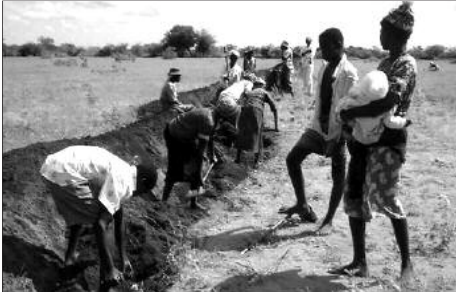
Contour ridge and infiltration pit under construction
