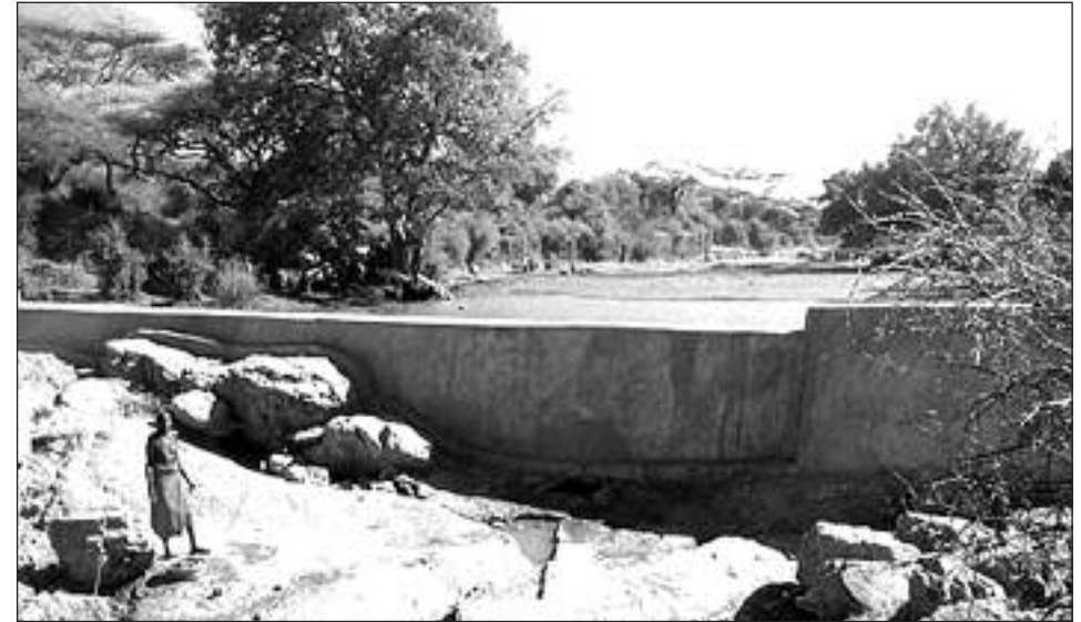
The completed dam after the rains
