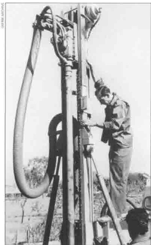
▲ Drilling for water in India in the 1960s. Oxfam financed several Halco Tiger rigs and British volunteers to supervise them and train local operators.
