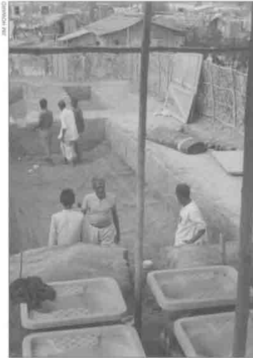
▲ Oxfam's Sanitation Unit was developed with help from the Universities of Surrey and Loughborough, with testing at the Cholera Hospital in Dhaka. It provides quickly-assembled facilities for large numbers and was used in the 1970s in refugee and squatter camps in Bangladesh.
