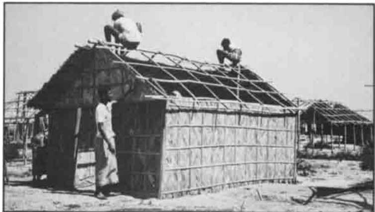
Figure 14. Plastic and bamboo matting house, Bangladesh
